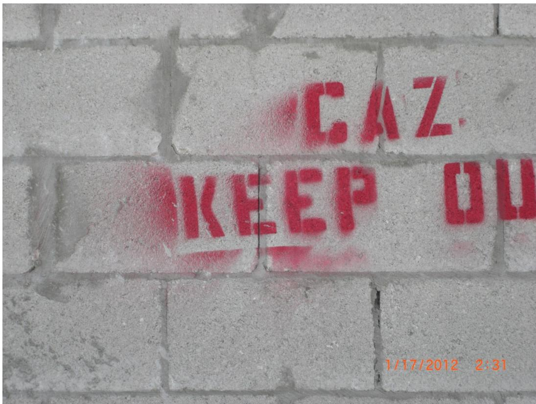
The crack above is due to mortar shrinkage. Sometimes these cracks will continue in a “stair step pattern following the mortar joint. Shrinkage cracks are very narrow (usually less than 1/32 inch) but will reflect through the stucco.
