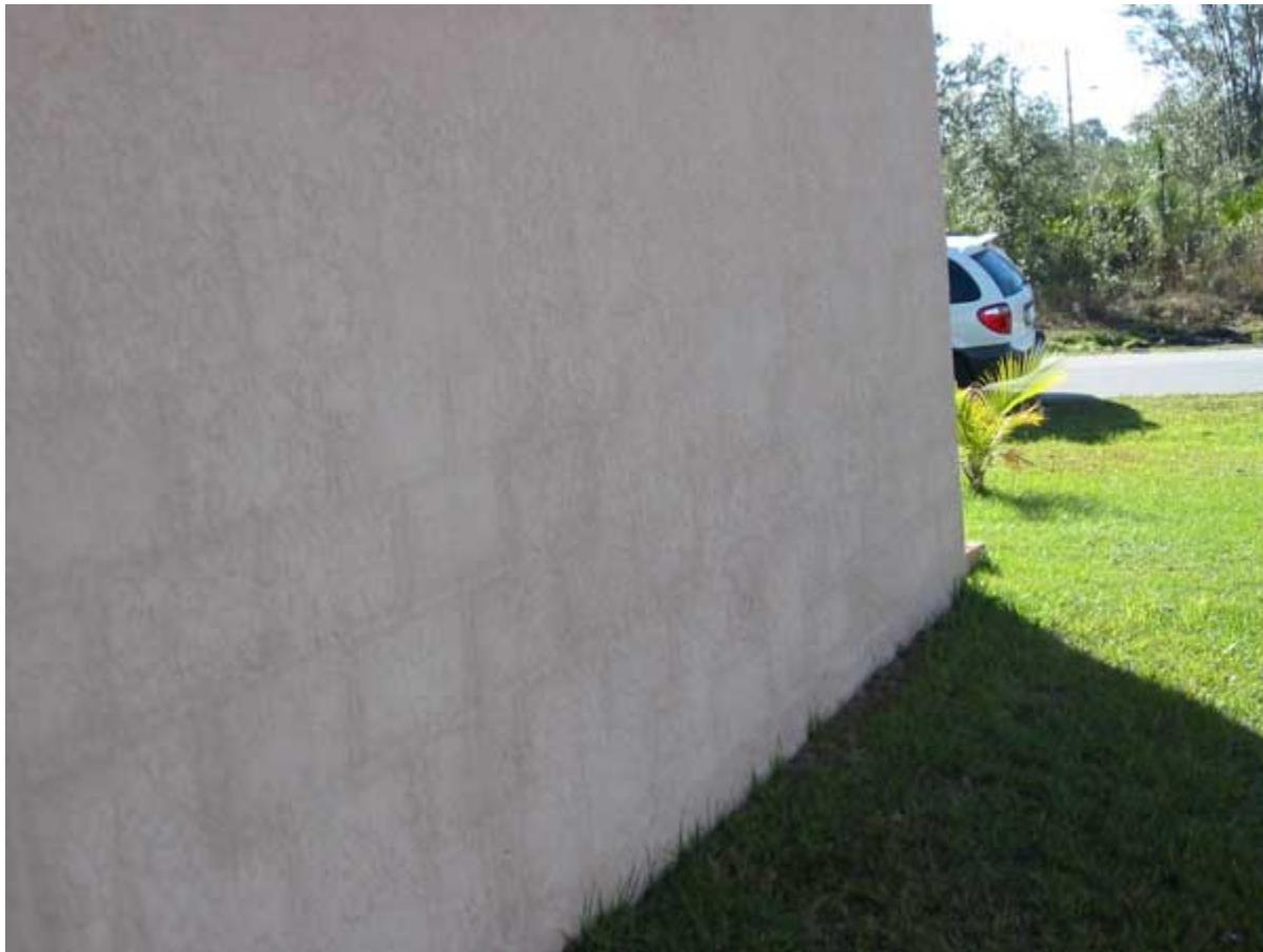
Factors affecting the ghosting phenomena include curing of the masonry wall, curing of the stucco and thickness of the plaster.
